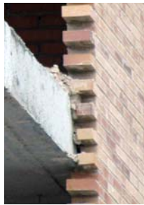
Figure.1. Traditional Spanish enclosure wall over-hanging on the edge of the floor slab.
