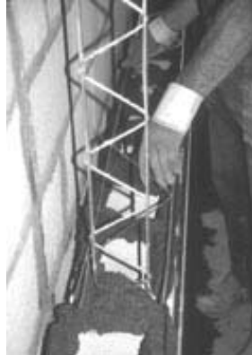
Overlap of right Murfor into AllWall rib
