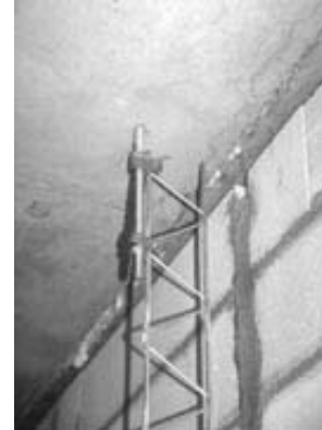
AllWall Telescopic fixing in the top of the rib
