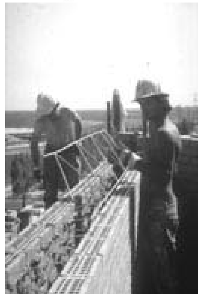
DCW Duplex Cavity Wall laying
