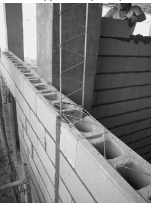
Murfor and AllWall rib only with mortar
