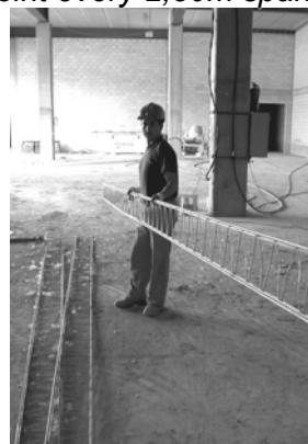
Easy manipulation of AllWall ribs h=8m
