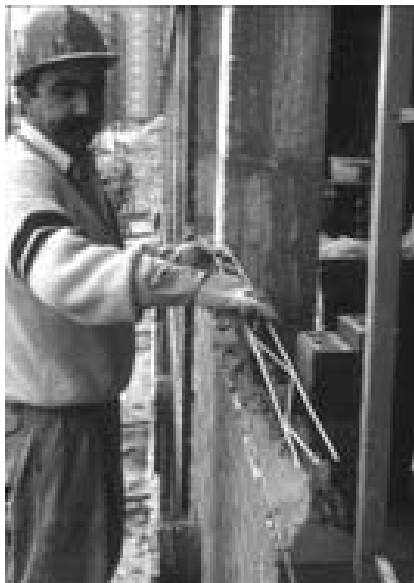
ACW Autosupporting Cavity Wall laying
