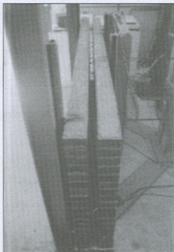
Figure 1. DCW Wall tied with Murfor bed joint reinforcement every 36cm high (6 courses).
