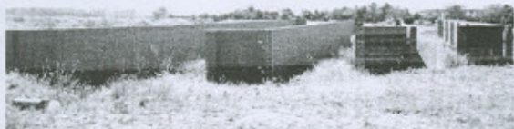
Figure 3. Base of the 1st course of Blockwork with Murfor.
