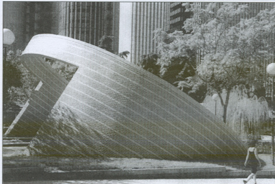
Figure 5. Convex side elevation of the Arch with brick courses set at 30°
