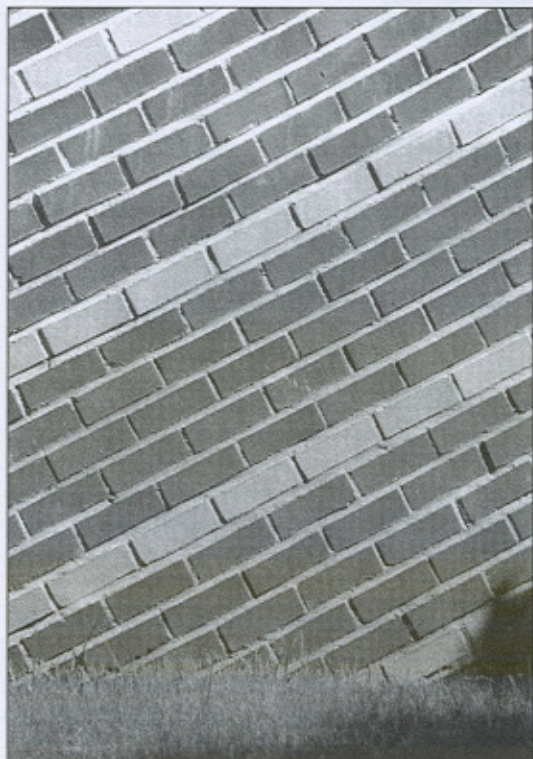
Figure 13. Detail of the concave external brickwork, with bed and vertical joints of standard thickness and pointed in mortar.
