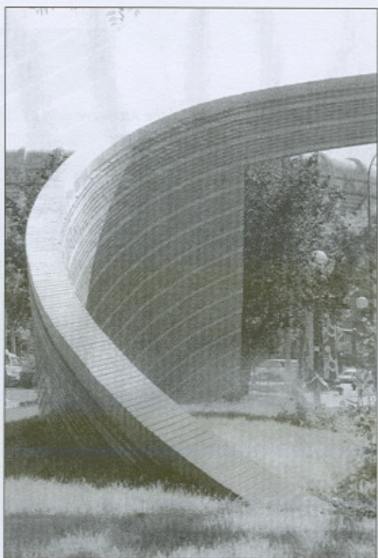
Figure 9. View of the concave and convex sections of the Arch abutment and its finial set in rowlock.
