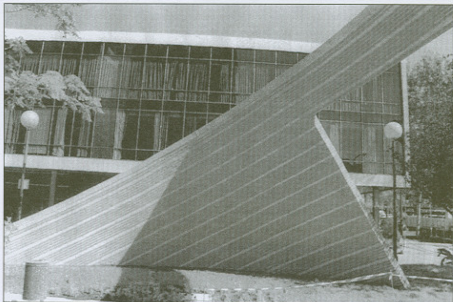
Figure 8. Internal convex view of the Arch abutments and 60° jamb
