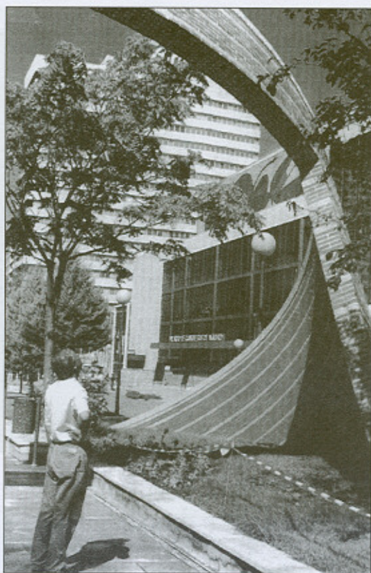
Figure 5. Convex side elevation of the Arch with brick courses set at 30°
