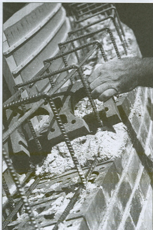
Figure 21. Placing of the laterally opened flower brick to receive the hoop
