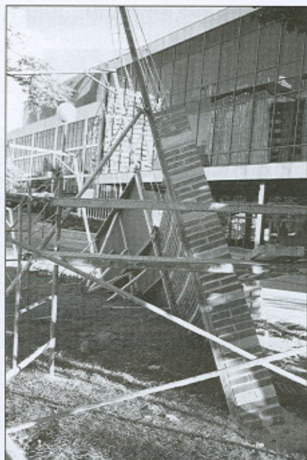
Figure 13. Springing of the one brick thick leaning jamb of the Arch in header bond at an angle of 60° to the vertical.
