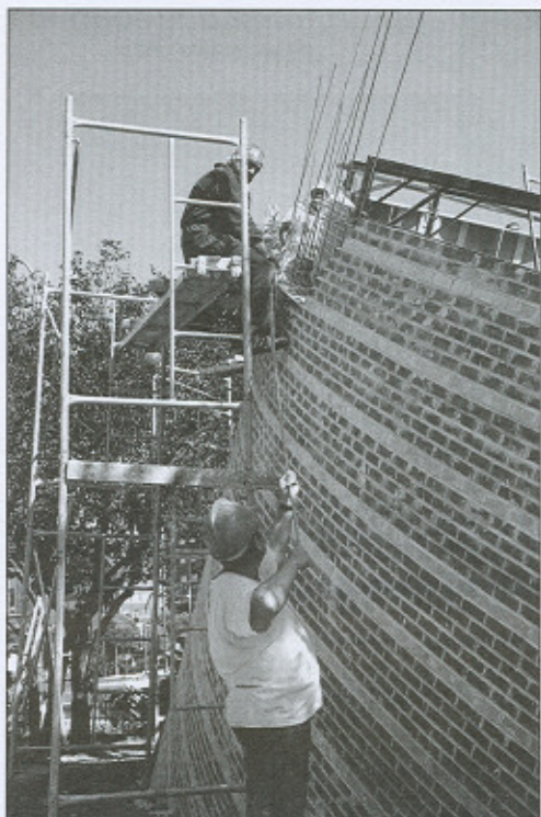
Figure 22a-22b. Laying of the continuous longitudinal bed joint reinforcement.
