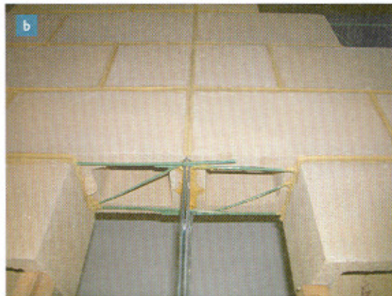
Fig. 9b Photo of the AllWall rib set in the continuous vertical joint of a wall at the Construmat '03 trade fair.
