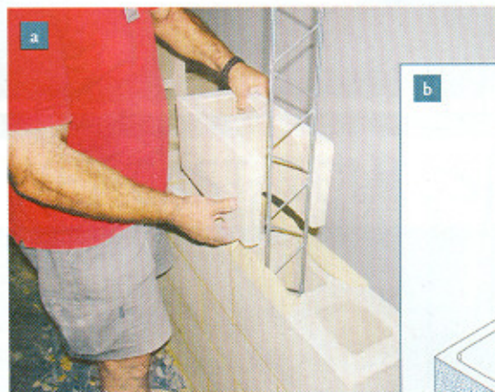
Fig. 4a Illustration of the sliding movement of the Bloc+ to house the AllWall vertical rib.
