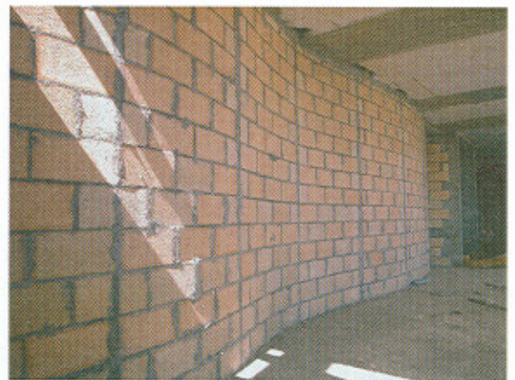
Fig. 15b 3 m high curved wall with rib reinforcement.
